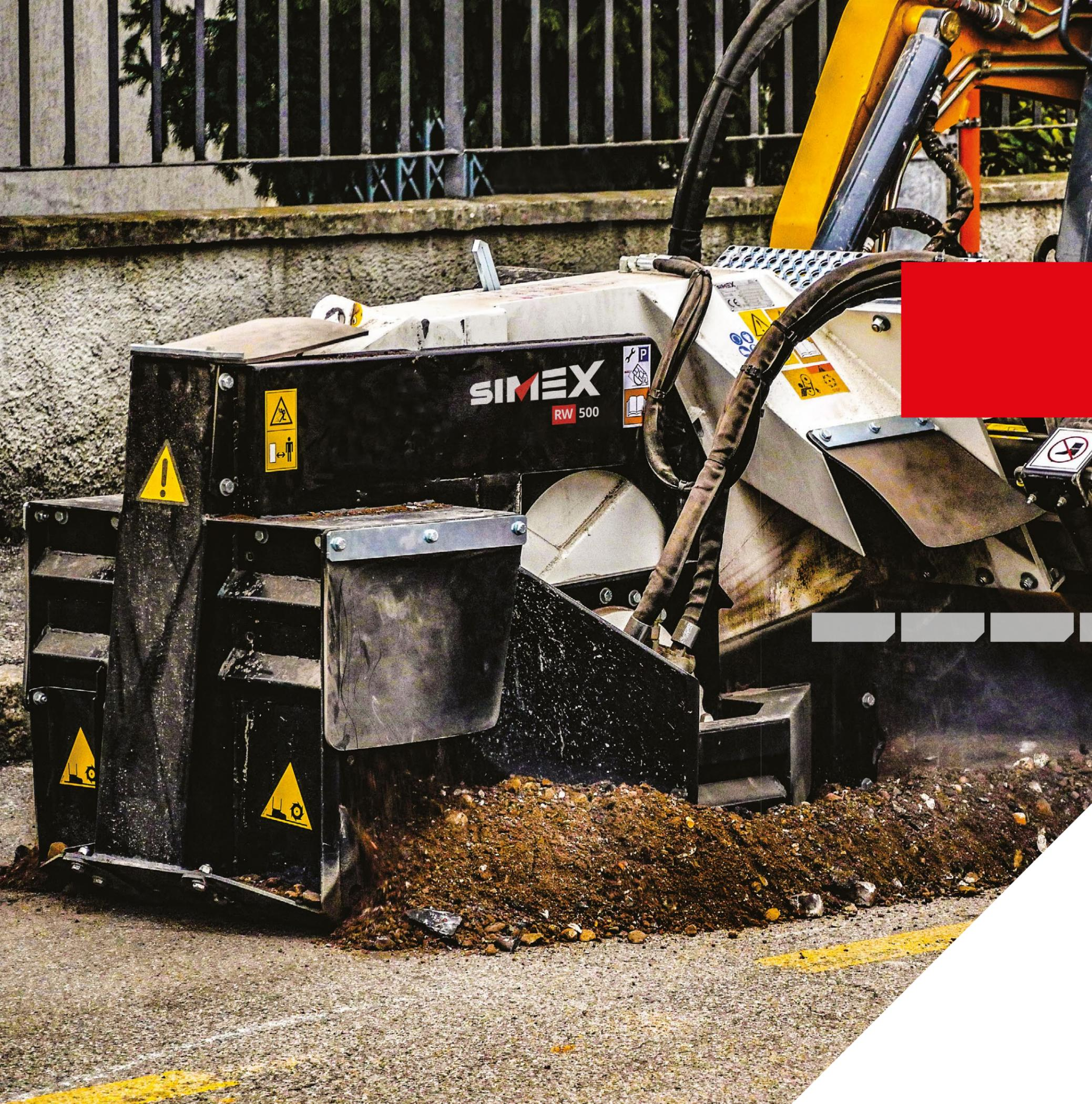
A large, black and white SIMEX RW 500 rock saw machine is shown in operation, cutting through a concrete surface. The machine is mounted on a yellow excavator. The background shows a metal fence and some greenery. The machine has several warning labels, including a yellow triangle with an exclamation mark and a yellow triangle with a gear icon. The SIMEX logo and 'RW 500' are visible on the side of the machine.
